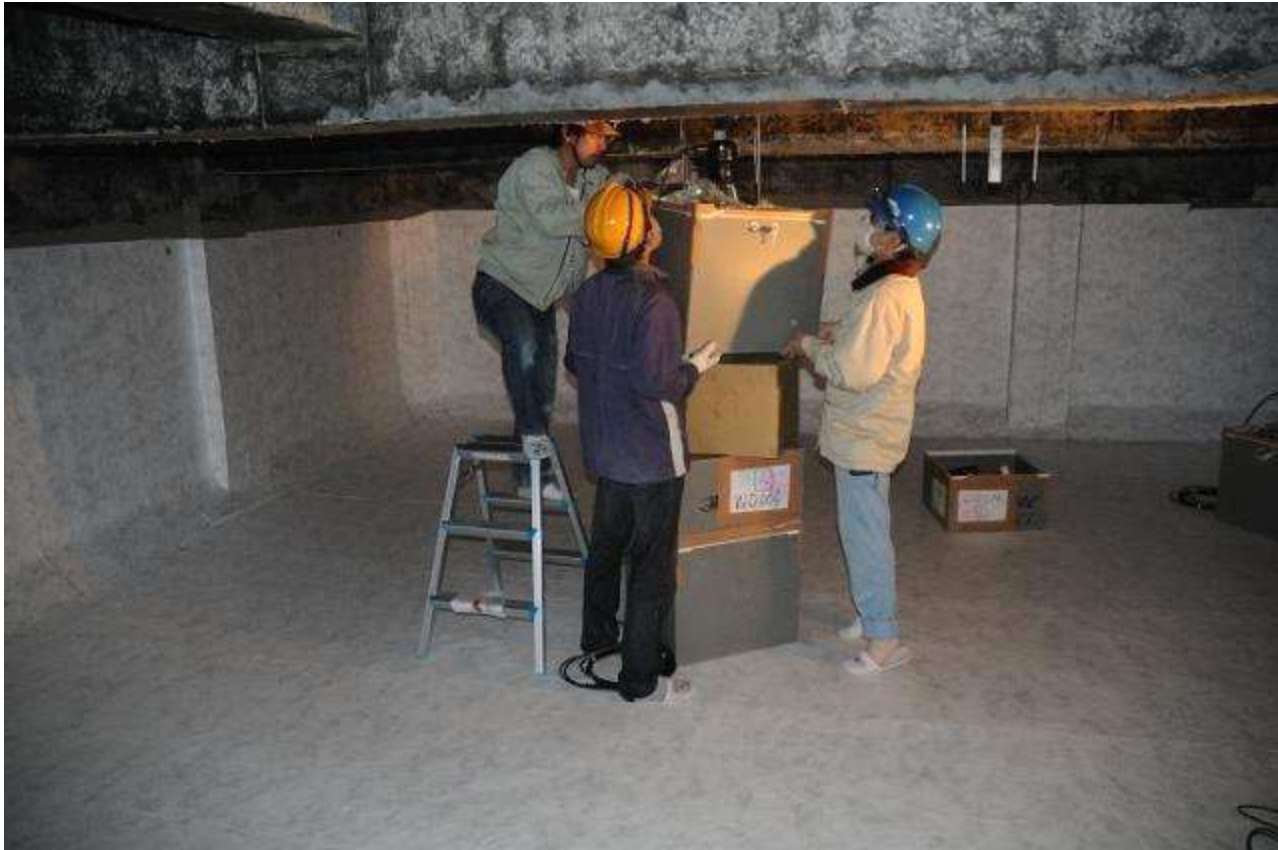
Installing a 20 inch PMT in a MD cell.
